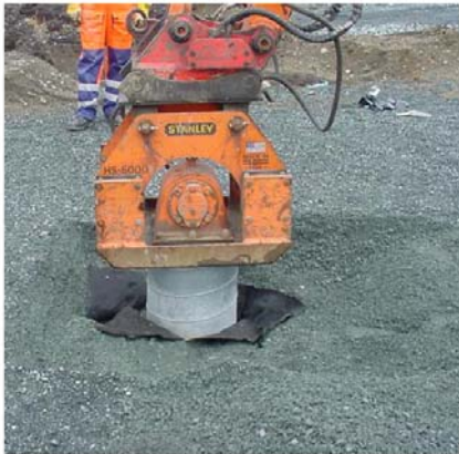
Figure 3. – Installing steel tube
