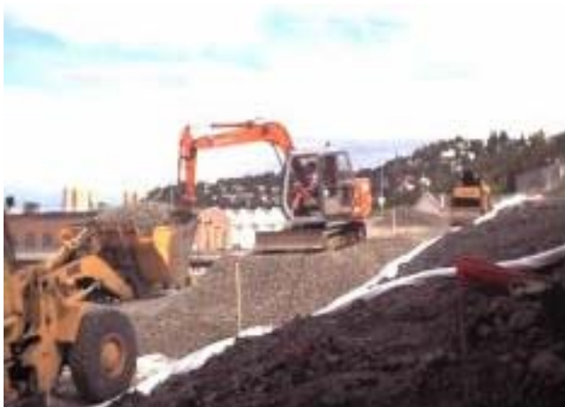
Figure 4 – Distributing foamglass using a crawler mounted excavator / shovel dozer
