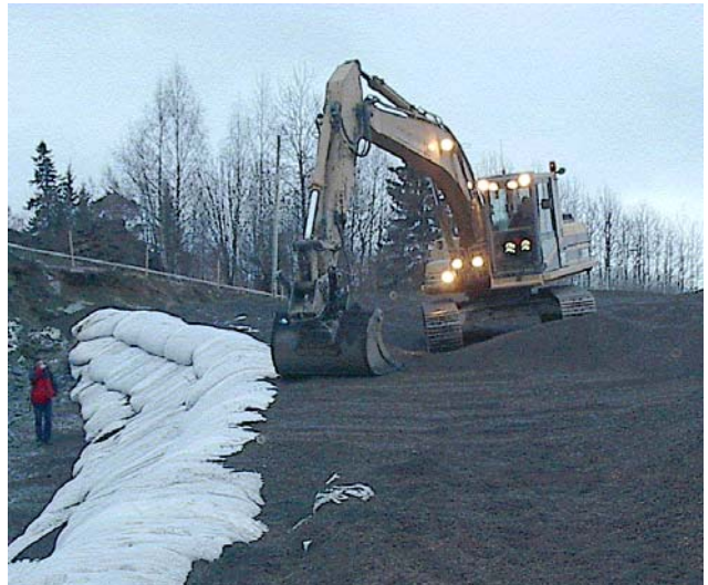
Figure 6 Digger laying LWA on the turned-up reinforcement
